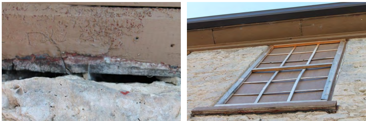
Figures 60 & 61 – (left) Detail, View of Building A, north elevation, second storey window sill and stone/mortar and exposure to the elements (right) View of Building A, north elevation, second storey window sill and stone/mortar (Source: MHBC, 2016)
