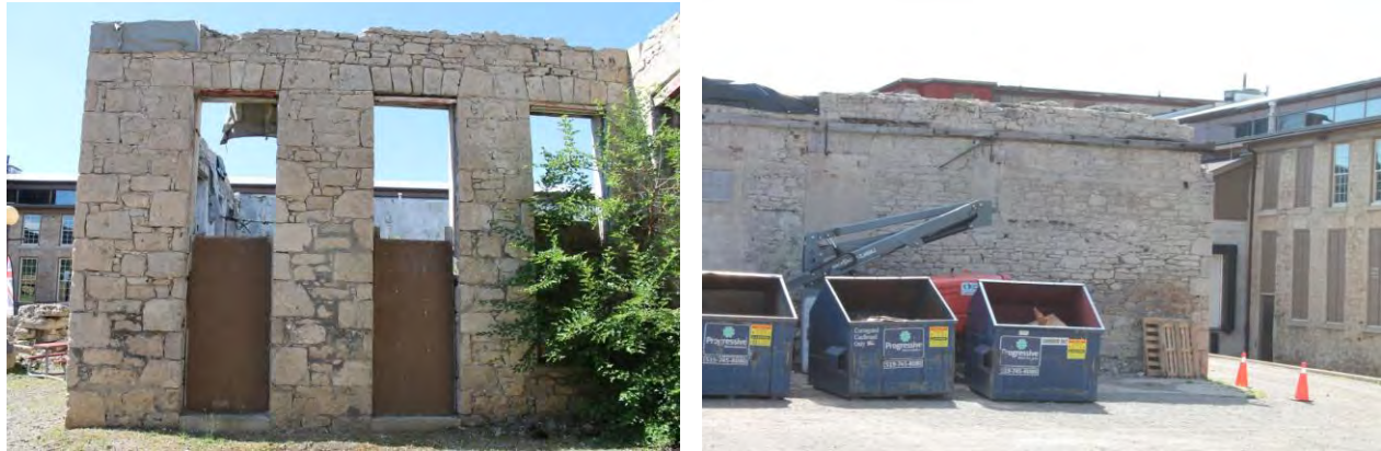
Figure 38 & 39 – (left) View of Structure E looking south. View of northern elevation partially boarded-up windows (right) View of Structure E looking east. View of western elevation stone wall with evidence of bricked-over window openings (Source: MHBC, 2016)
