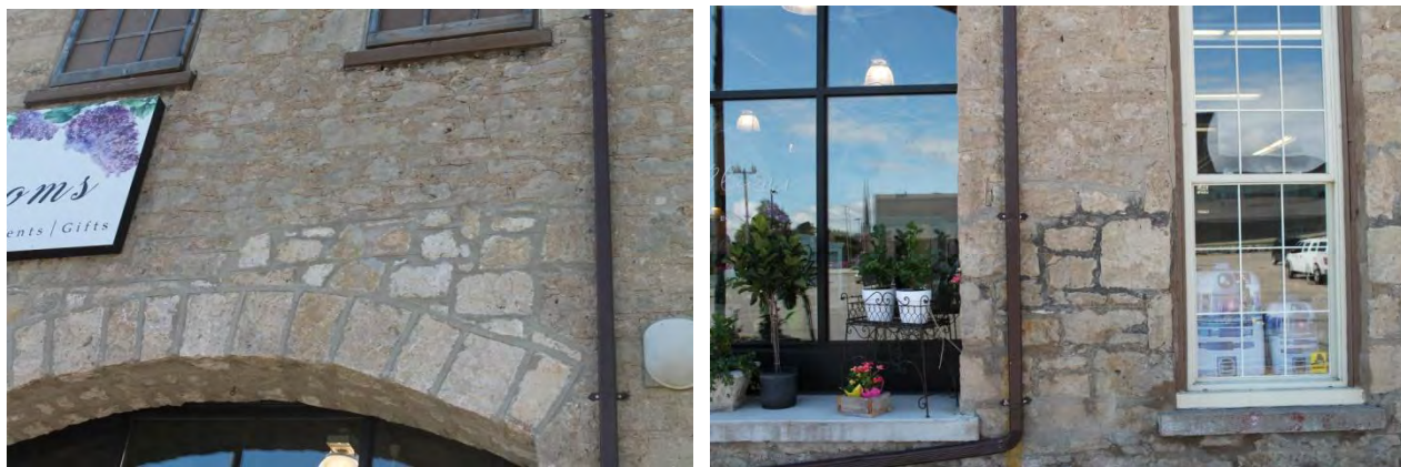
Figures 58 & 59 – (left) View of Building A, north elevation, detail of masonry repair (right) View of Building A, masonry repair (Source: MHBC, 2016)
